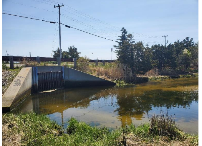
Upstream trash rack near low tide – Photo taken May 2023
