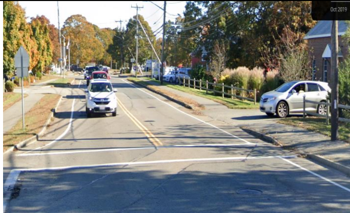
3 Low-visibility crosswalk and missing sign
