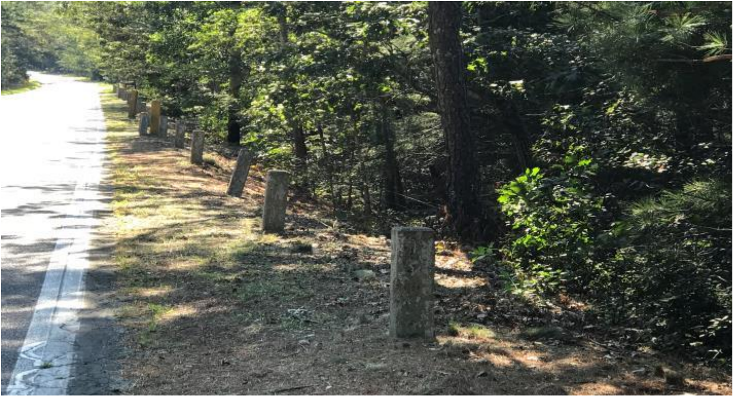
Concrete Guardrail Removal
