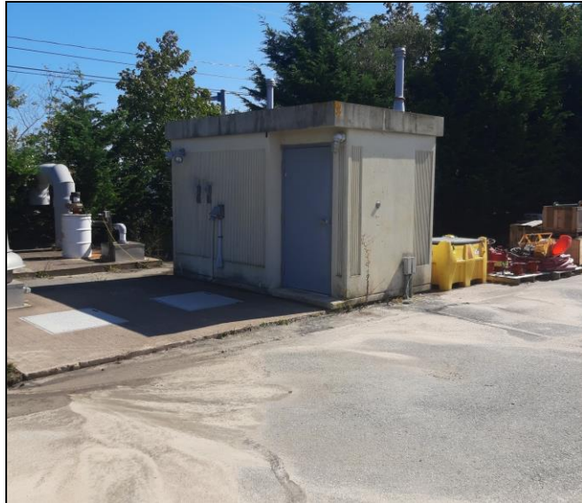
Photo 4: Bearse's Way Pump Station Exterior
