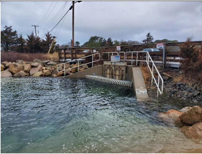
Tide gate near high tide – Photo taken March 2023
