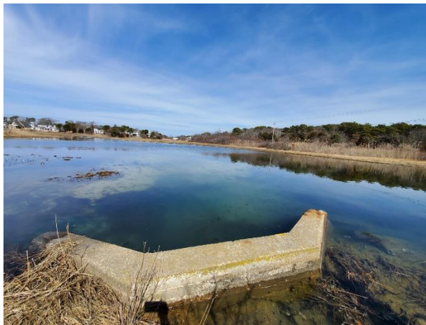
Culvert headwall and up-gradient salt marsh (taken 3-15-22).
