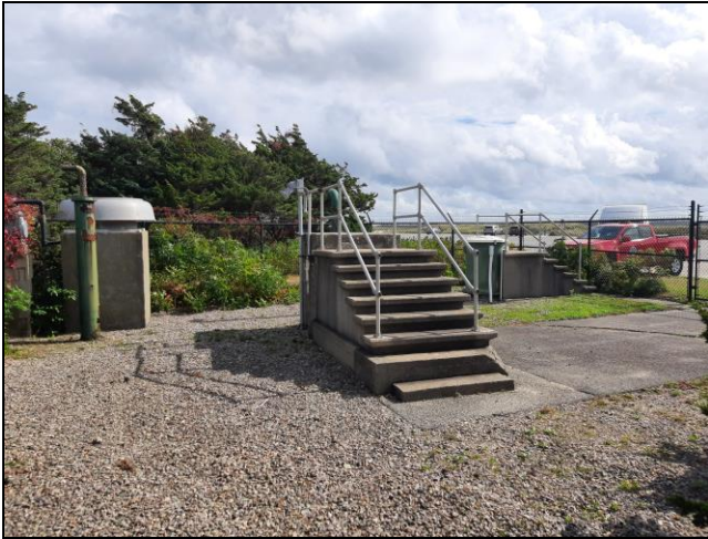
Photo 1: Kalmus Beach Pump Station
