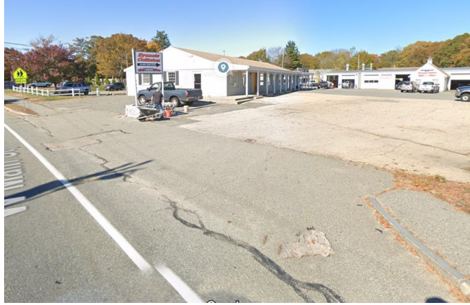
1 Example of excessive driveway opening
