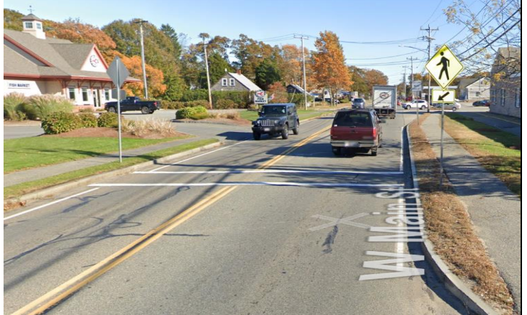
2 Example of crosswalk missing curb ramps
