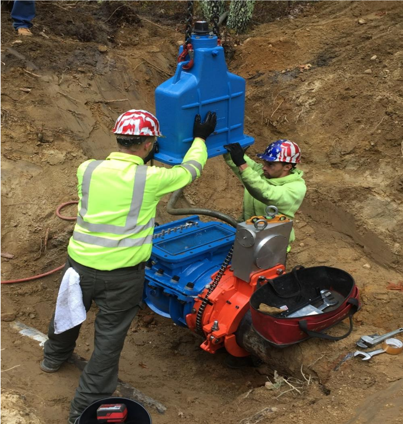
Pipe Replacement Project-2023
