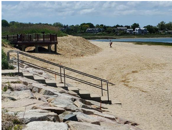
Close up of Post Nourishment with high tide line staked, indicating a narrow work area between the toe of the dune and the high tide line. Also, the high tide line extends up to and within the toe of the adjacent private stone revetment. Picture taken May 2022.
