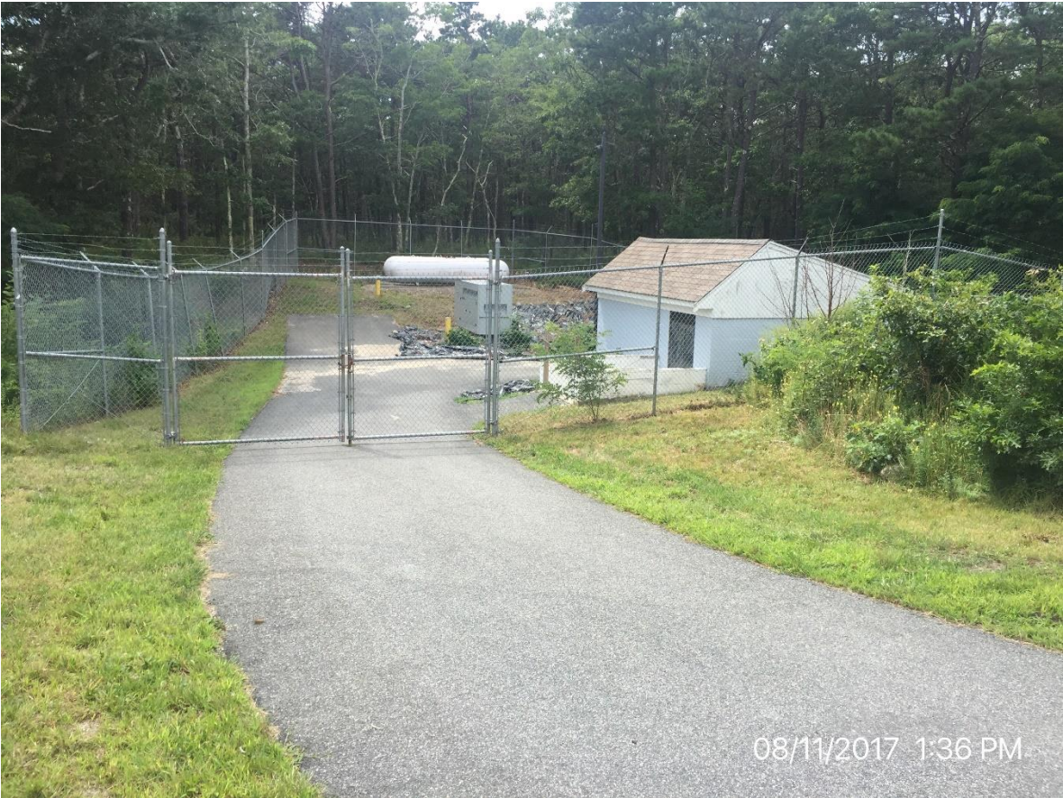
Water Pump Station
