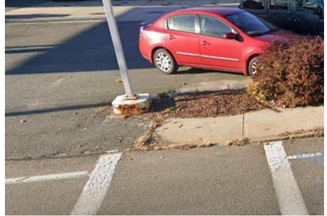
Missing detectable warning
